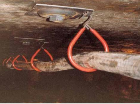
Versatile CAB Cable Clips safely suspend all types of electrical cables.
