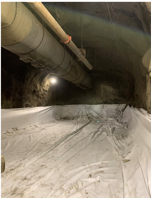
Dewatering Bag Setup
