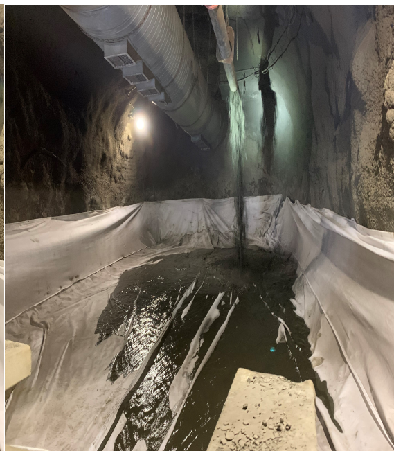
Dewatering Bag Filling
